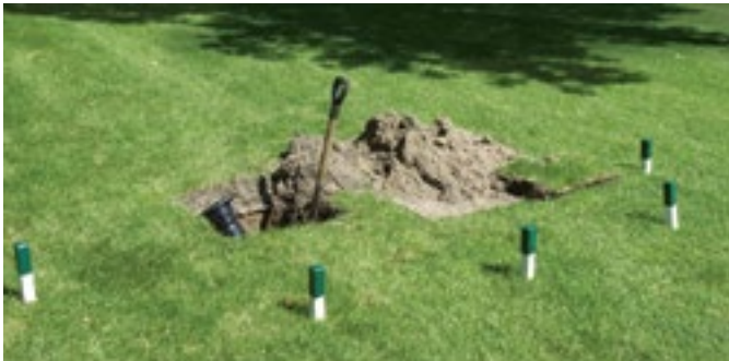
Mark off repair areas.
